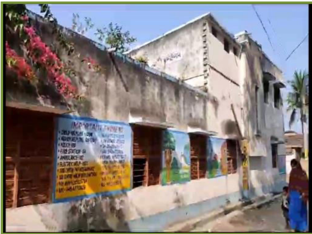
SCHOOL WALL PAINTING
